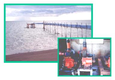
A complete hatchery with 100 breeders requires a set of two water pumps of four-inch diameter water pipe running 24 hours. Another set maybe required as alternate or backup units. A satellite hatchery (without breeders) will require just one unit of pump, preferably a diesel-run unit like Kubota or Yanmar.
